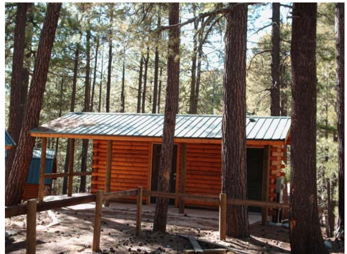
Restroom & Shower House Accompany the 5 cabins
