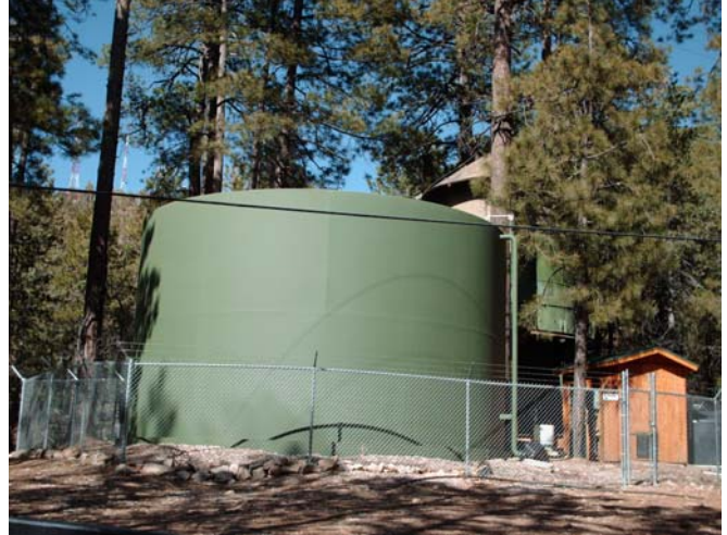
1 of 5 Water Tanks Water storage capacity exceeds 120,000 gallons
